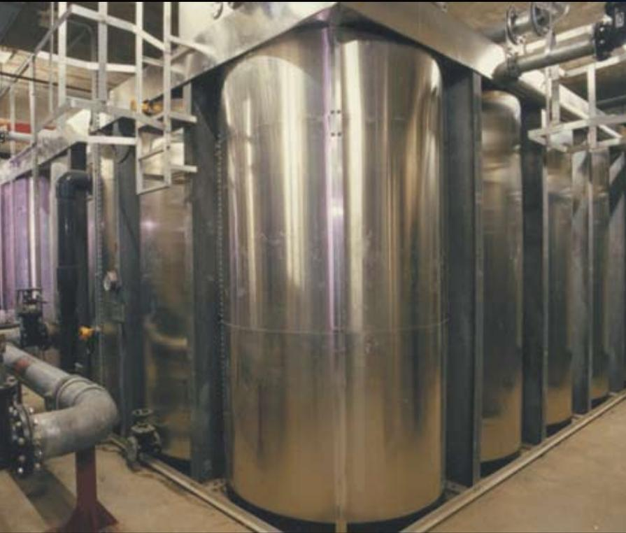
Where space is at a premium, the Liquitainer<sup>®</sup> / Firetainer<sup>®</sup> tank is an ideal solution for bulk water storage indoors or out. A wide range of shapes and any length or width can be catered for, with a maximum height of 5.35m in galvanised and aluminium.
