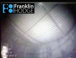
Underside of tank cover
