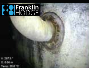
Overflow pipe & connection
