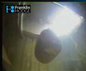
Inlet valve ball float
