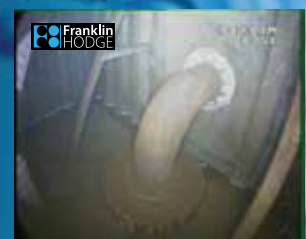
Tank floor area & fittings
